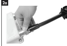
Connect the 1/2" connector to the device port and hand tighten. Device port must be free of tar, butyl, and vinly tape residue before beginning this step.
