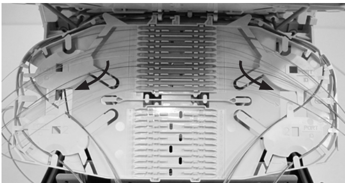
9.5.6. Always start with splicing the fibers of area 1. Make fusion splice per standard practice and push the splice protector (SMOUV 45) in the splice holders starting with position 1 (top position). Install the fibers in the correct color code sequence if required.
