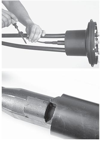
3.7.4  $\,$  Tighten the trigger until it butts. When necessary, use wrench (n° 12) to tighten the trigger.
