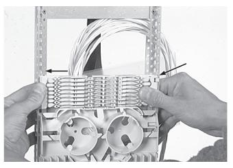
3.9.3 Fix the wraparound groove plate on the UMS by putting the plate with the long protrusions in the S1 UMS-profile and sliding the plate in the S2 UMS-profile until it snaps. (Do not leave gaps between groove plates).
