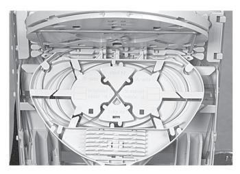
3.9.10 Store the fibers temporarily on a tray (the picture shows the case of a loopback).
