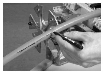
3.6.1 Guide the cable without torsion to the desired port and mark the cable. This line is used to position the cable retention device. See next steps.
