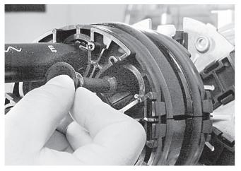
3.7.2 Before closing the gel block make sure it is clean. Insert the plugs in the unused ports.
