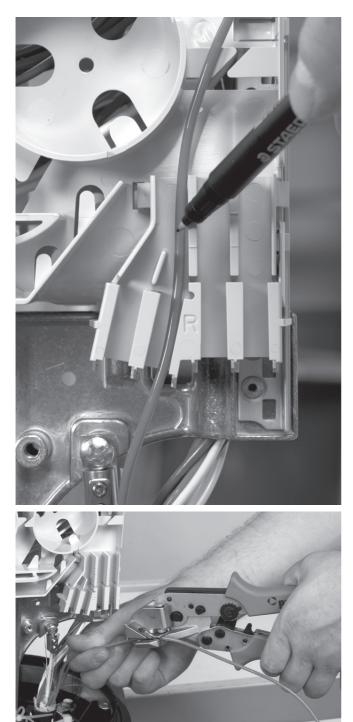
3.8.3 **In case of reversed oscillating cable**: separate the loose tube(s). Match the loose tube(s) on the tubeholder and mark both sides between the two marks. Shave between the two marks with the appropriate tooling.
