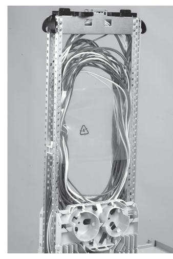
3.8.1 Remove the plastic parts at the top and the sides of the UMS profiles. Make some loops with the uncut loose tubes and put these in the plastic bag (be careful not to damage the loose tubes!). Two sizes of bags are available. Use the correct size according to the volume of the loose tubes. If needed use two bags. Slide the bag between the UMS as shown. Close the UMS.
