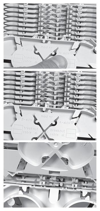
3.9.5 Place a tray in the wraparound groove plate: do this by pushing the lip on the groove plate slightly up with the tray and move the tray laterally into the hinge cavities. Start from the FAS block side and preferably mount trays as you fiber up. In case of SC trays do not leave spaces. In case of SE trays always leave one hinge facility open (between that FAS block and tray or tray and tray).
