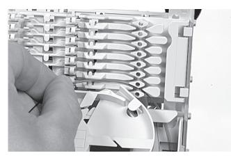
3.9.8 Route the fiber in the correct groove of the wraparound groove plate to the entrance of the identified tray. Fiber must be routed in the groove behind the hinge of the tray!
