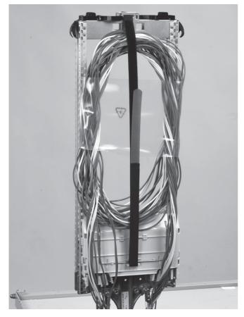
$3.12.2\,$  Make sure the two foam blocks are on top of the UMS profiles.  $\ensuremath{\textbf{Note}}$  : the foam blocks have a functional purpose.
