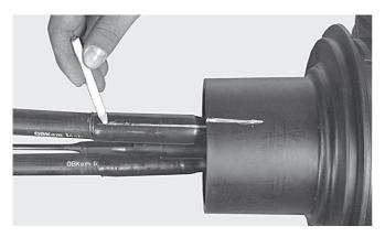
3.7.5 Mark base and cable (see picture). **Note**: these lines on base and cable must always match when the closure is moved.
