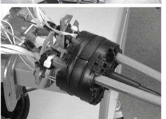
3.7.1 Remove the protection of the gel block and open the gel block. Position the open gel block in between the cables. Leave  $\pm 2$  cm between the gel block and the cable attachment plate.
