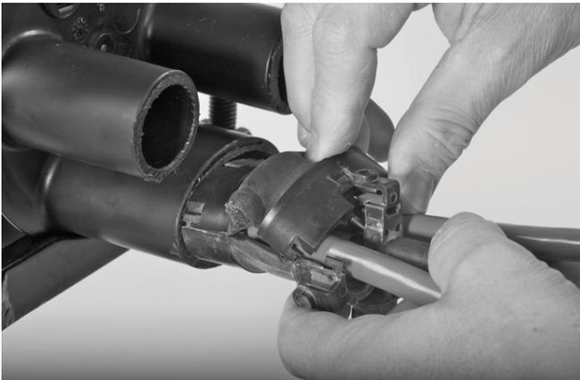
3.4.4 Take the first gel part (with trigger) and put the cables in place, if needed (when large cables) lubricate the cables. Take 2nd gel part and insert the pins in the corresponding holes at top and bottom. Push till snap fit (click).
