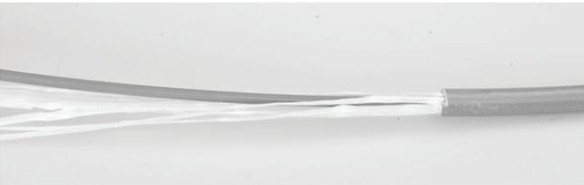
3.5.5 Remove 1.3 m of jacket and cut strength member at 40 mm.
