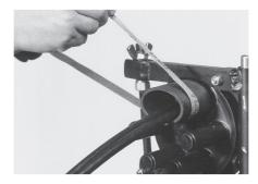
6.3 Place oval seal over the oval port and cable. Mark the sleeve length onto the cable.
