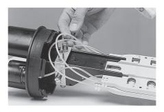
16.5 Carefully bend the intertray jumper tube to the appropriate tray and secure to the splice tray with two tie-wraps.
