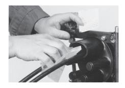
6.2 Abrade oval port and cable sheath circumferentially on the cleaned area with the abrasive strip. Remove any abraded material with a clean cloth.
