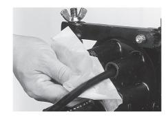
11.7 Abrade port and cable sheath circumferentially on the cleaned area with the abrasive strip. Remove any abraded material with a clean cloth.
