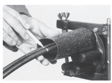
6.4 Match the blue line of the aluminium cable protection foil with the marks on the cables. Wrap aluminium cable protection foil around cable.
