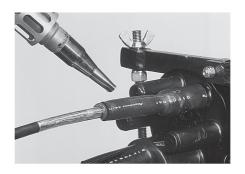
11.12 Wait until the sleeve is cool to the touch before moving the cables.
