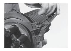
4.2 Install the FOSC in the FOSC-STAND and open the oval port for cable entry by cutting the port at the ridge with a hacksaw. Deburr the inner edge of the port opening with abrasive strip.
