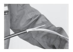
5.2 If a shield continuity is required, cut cable sheath axially for 25 mm from cable ring cut. Crimp shield clip on cable sheath with pair of pliers.
