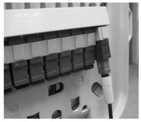
10.6 Remove the drop cable dummy rods
