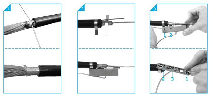
16.2.1 Remove 20 mm of the cable jacket to clear the metal layer, if present. A nylon wire can be used to prevent damaging this layer. Verify that the metal surface is as smooth as possible and sand carefully just to remove the coating. Make sure the metal layer is not damaged.
