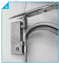
9.3.3.4 Secure the jacket of the cable to the CTU by first tightening the screw on the side and then tightening the screw at the back side of the CTU.
