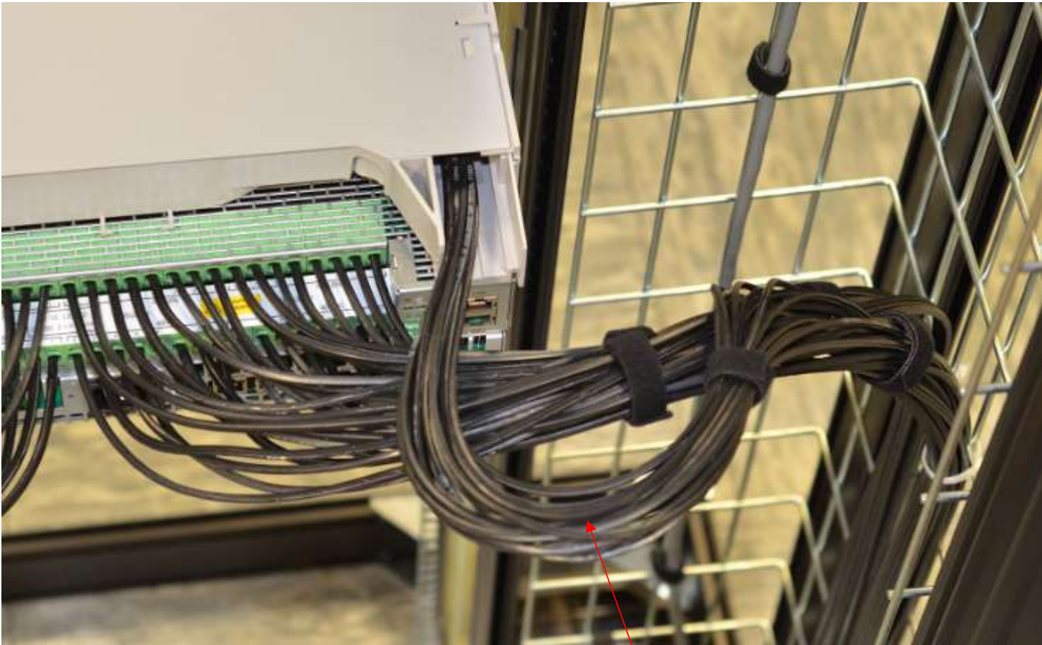
When installing fibre always allow sufficient service loop for fibre tray removal.
