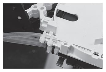
2.8 Secure the transportation tube with two tie-wraps.
