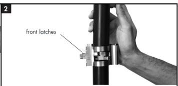
The installer might need to push the hanger onto the cable (away from the open end), to facilitate closing the front latches.
