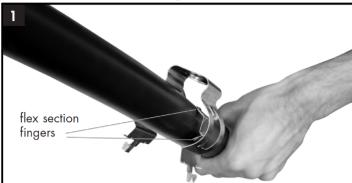
Position hanger onto the cable. Ensure four fingers of the flex section are on the cable. **NOTE: Make sure cable is straight.**
