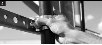
The front latches of the hanger should be squeezed to fit into the  $\frac{3}{4}$ " hole.
